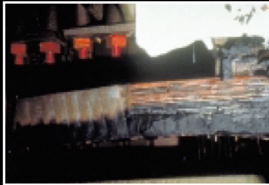
[2] Geomagnetically induced current (GIC) caused highly localized, although severe, damage to this large step-up transformer in a mid-Atlantic U.S. state in 1989.
